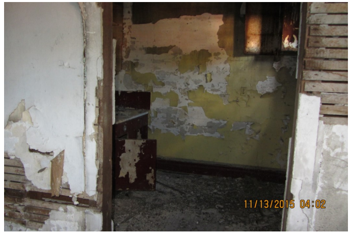
Third Floor Interior
