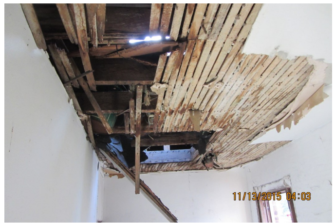
3rd floor ceiling
