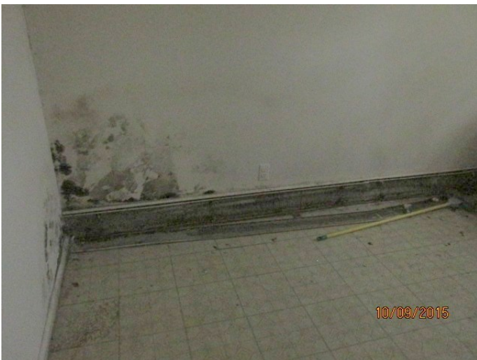
Interior photos showing water damage
