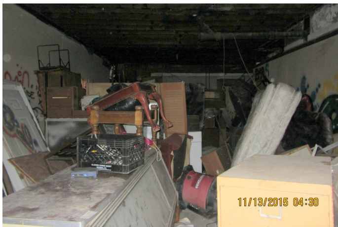
1st floor—Former retail space
