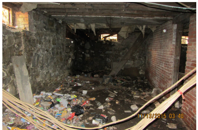
View of the basement
