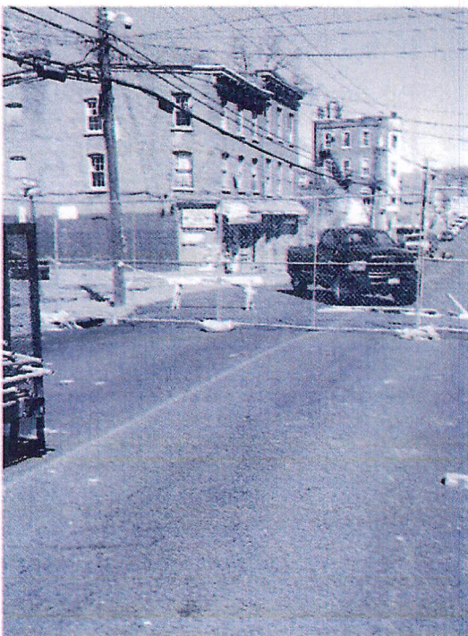
Temporary Fence Constructed – Approximatley 35' Wherever Practicable
