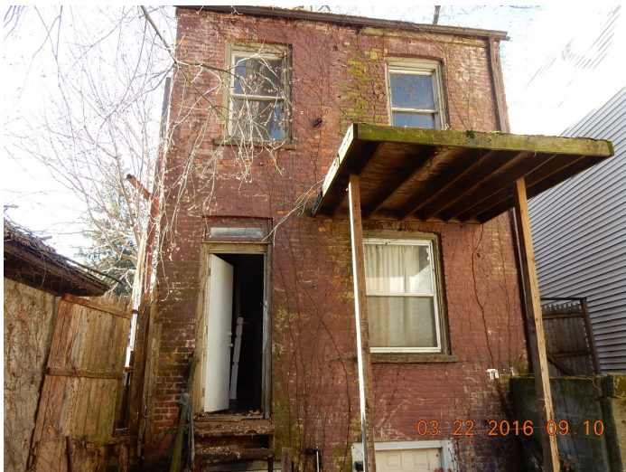
Rear of house
