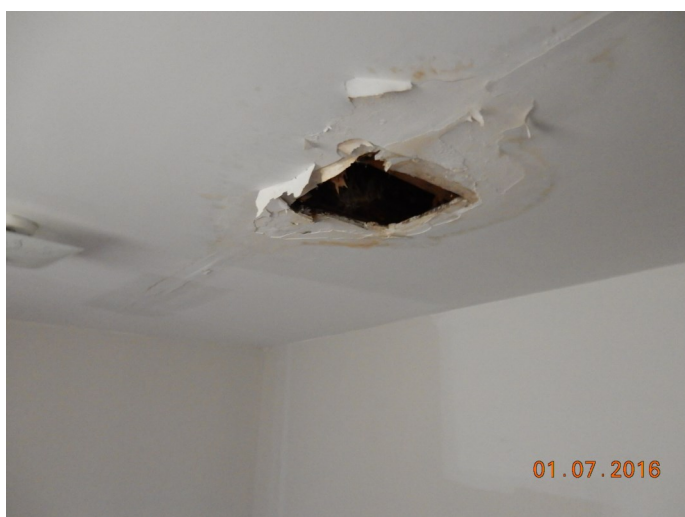
2nd Floor Ceiling Leak Marks
