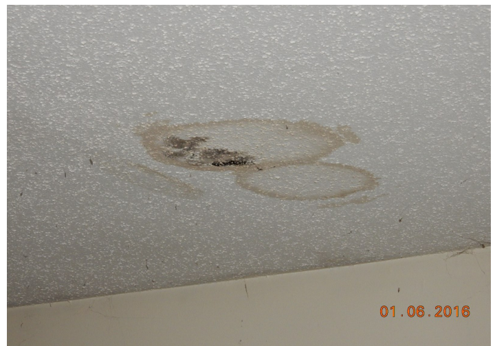
2nd Floor Ceiling Leak Marks
