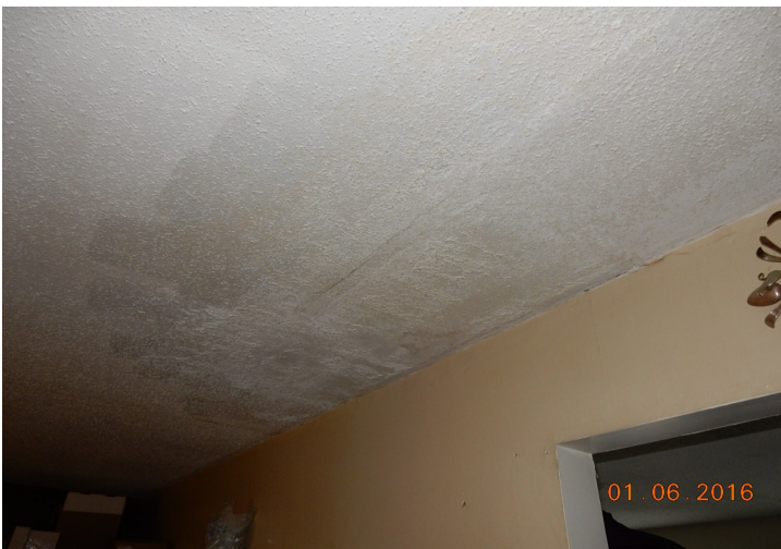
2nd Floor Ceiling Leak Marks
