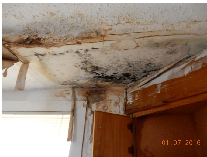
2nd Floor Ceiling Leak Marks
