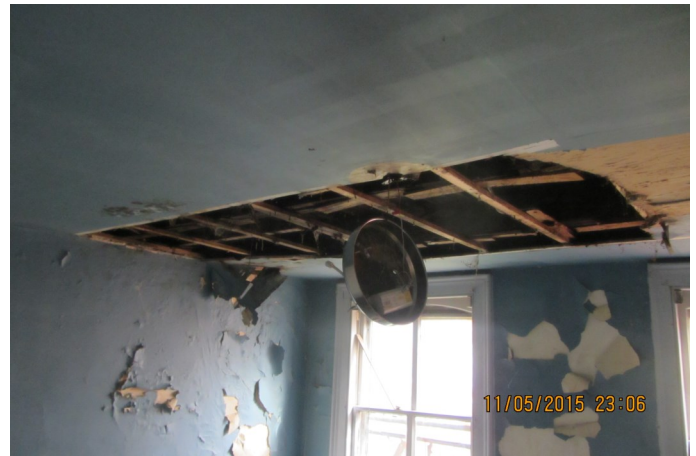
3rd floor ceiling
