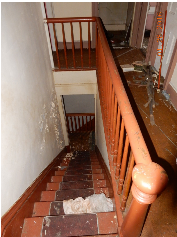
Third floor stairwell
