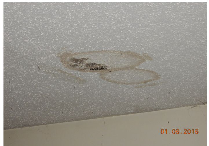
2nd Floor Ceiling Leak Marks
