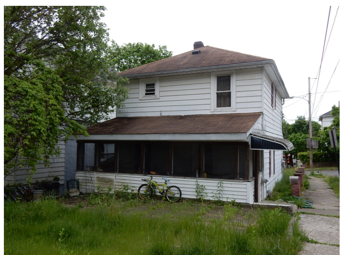
Rear of House
