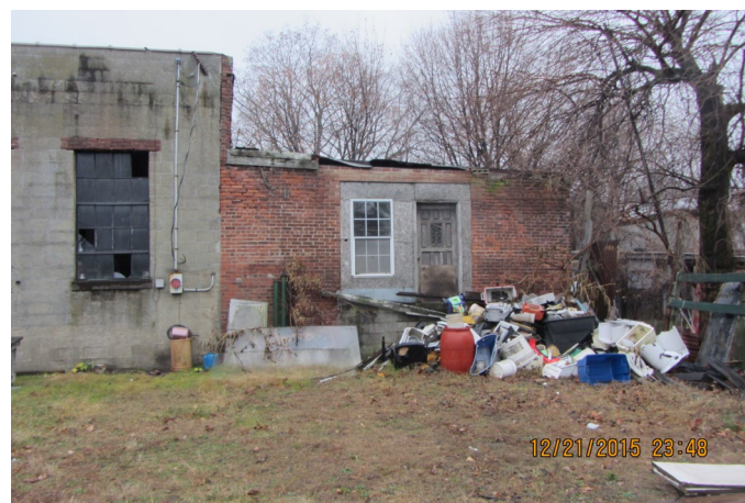
Exterior of the side building.
