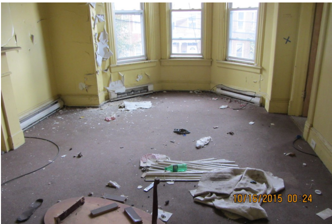
2nd floor room
