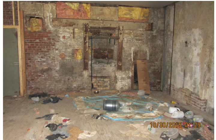
1st Floor Commercial area
