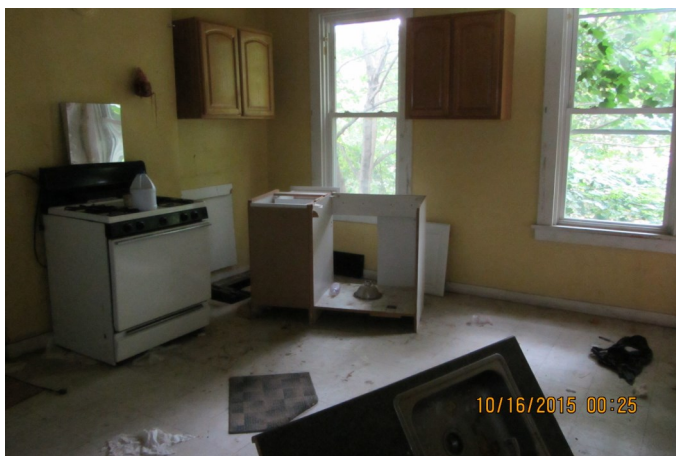
Second floor— kitchen
