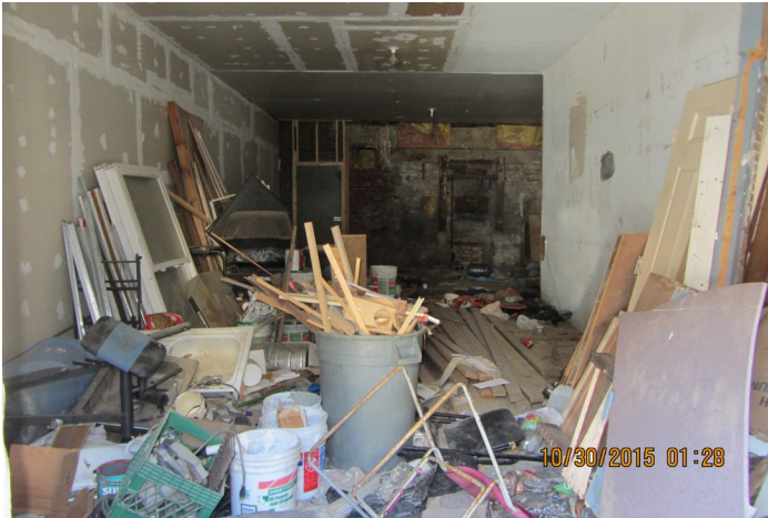
1st Floor Commercial Area
