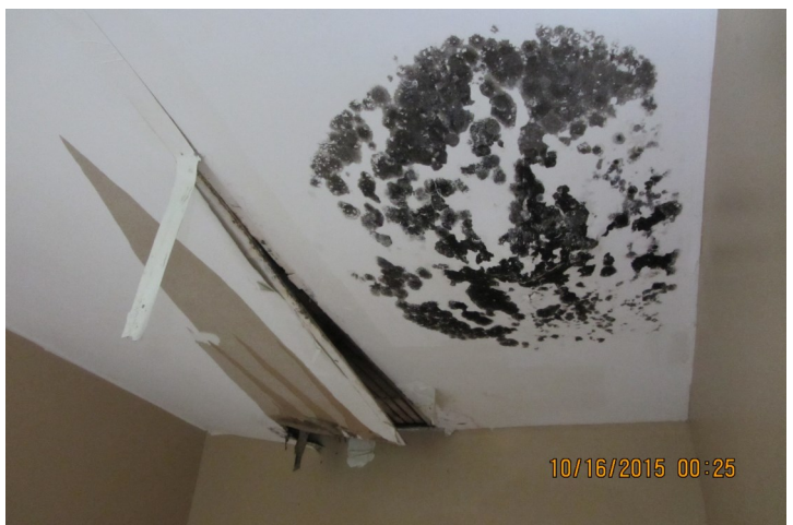
2nd floor ceiling
