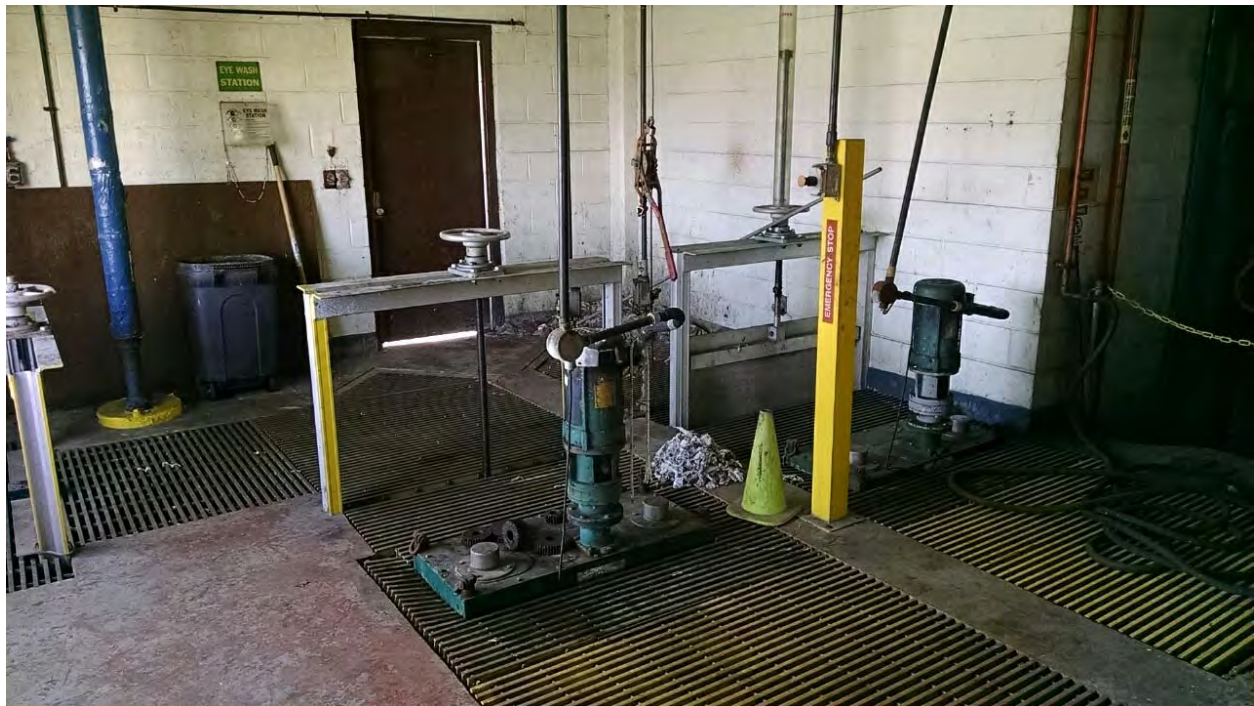
Photo 4 – Interior of Screenings and Grit Removal Building
