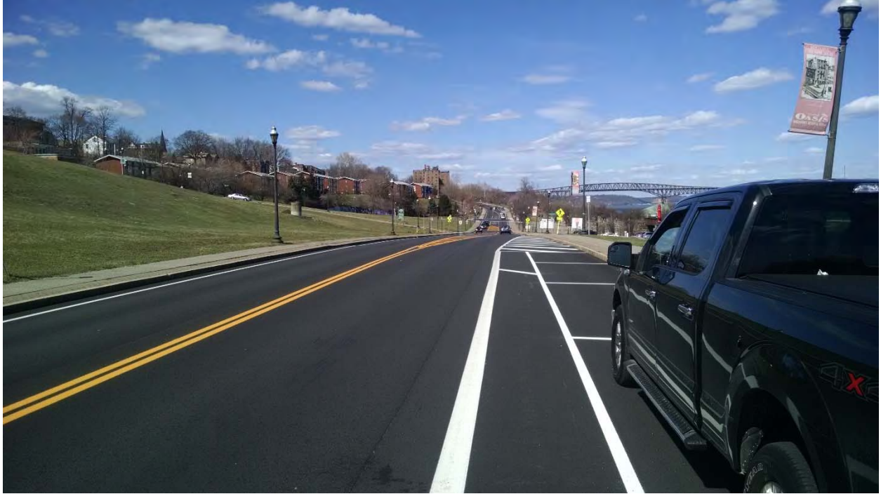
Photo 3 – South Water Street @ First Street looking north
