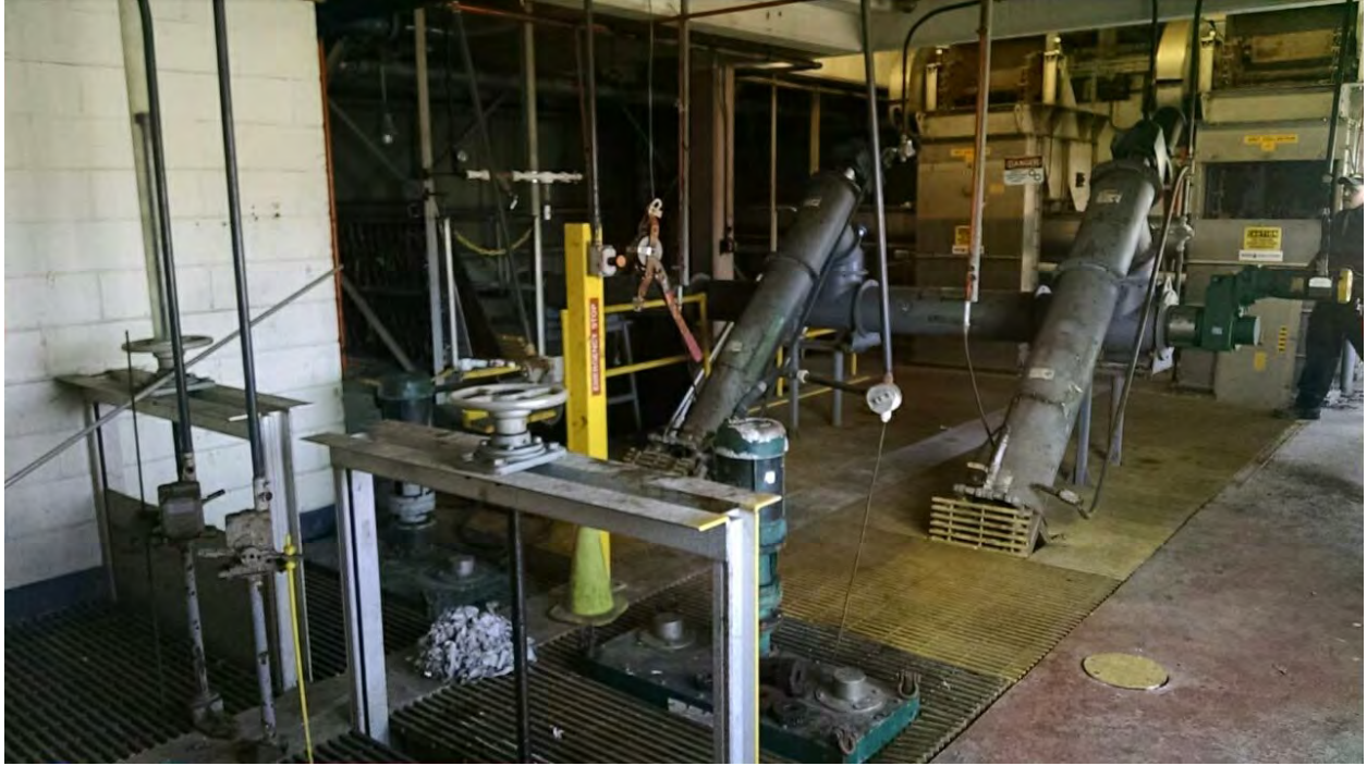
Photo 5 – Interior of Screenings and Grit Removal Building
