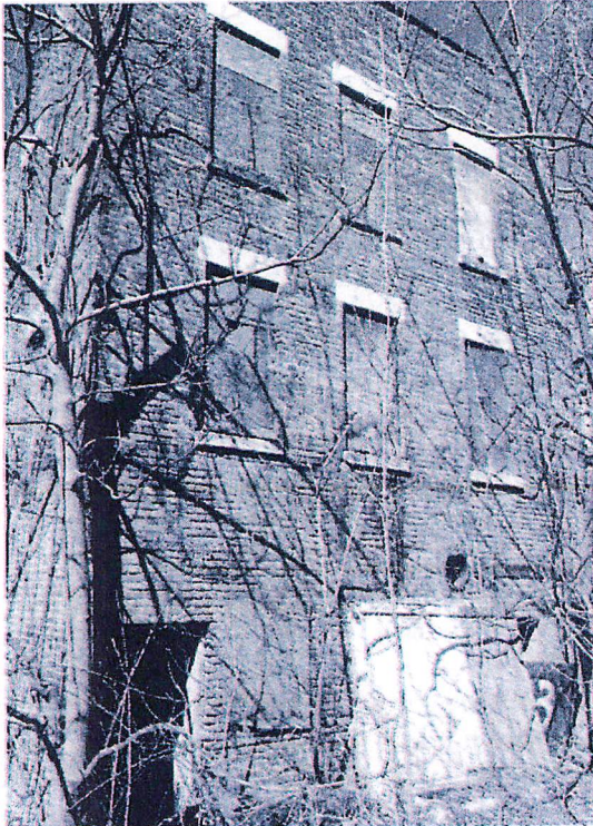
Exterior South Façade – Intact (Typical)
