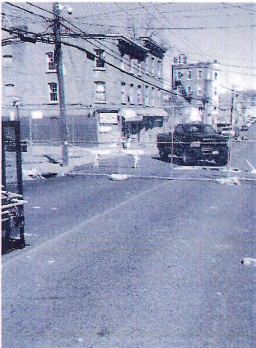
Temporary Fence Constructed – Approximatley 35' Wherever Practicable
