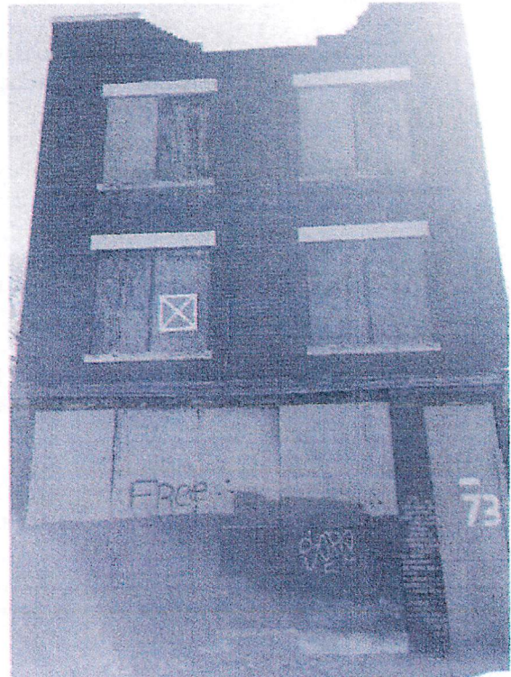
Exterior West Façade – Intact (Typical)
