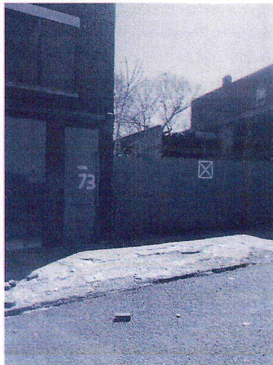
West Façade, Including Adjacent 77 William - Approximatley 20' Away
