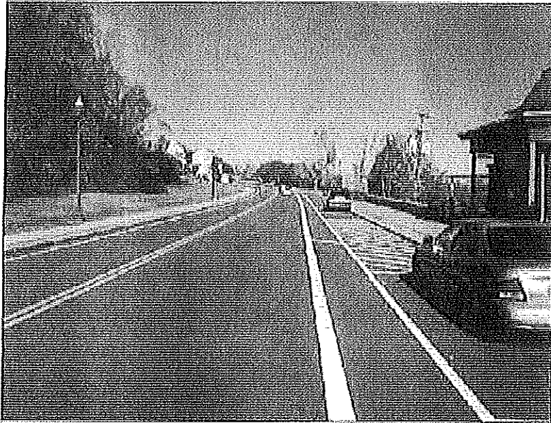
WATER STREET LOOKING NORTH
