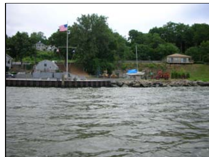
26 – Steel sheet pile bulkhead
