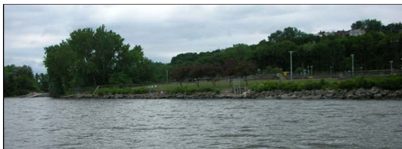
7 – Riprap shore protection
