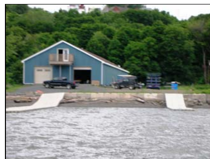
6 – Concrete block bulkhead
