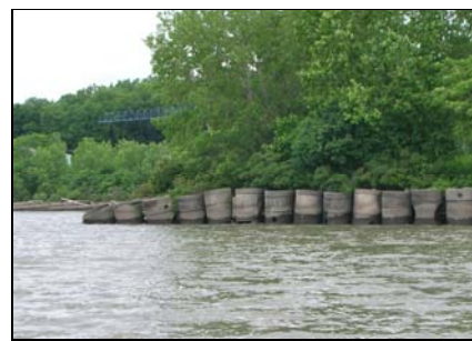
4 - Stacked concrete rings
