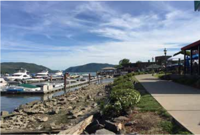
10. Riverfront Walkway and Riverfront Marina looking south.
