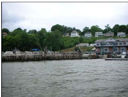
25 – Timber pile breakwater
