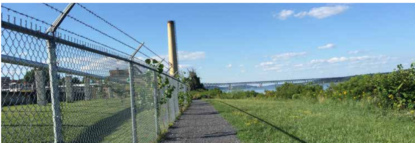
18. View of Waterfront Trail and Water Pollution Control Plan looking north.
