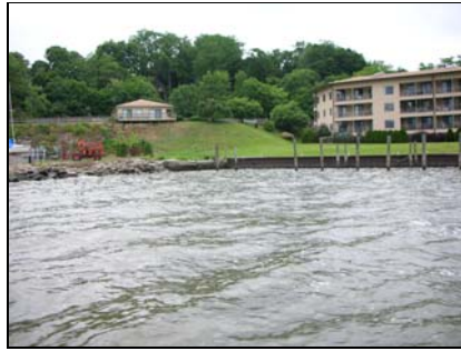
27 – Steel sheet pile bulkhead
