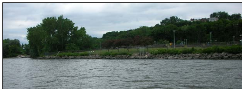
7 – Riprap shore protection
