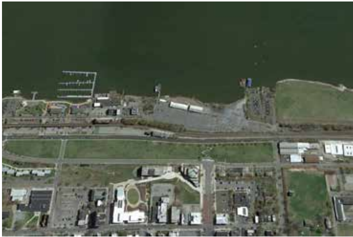
13. Aerial view of central LWRP area and vacant development sites.
