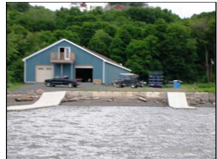
6 – Concrete block bulkhead
