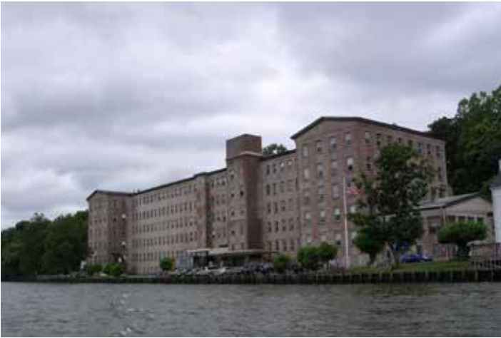
4. Regal Bag property from Hudson River looking south.
