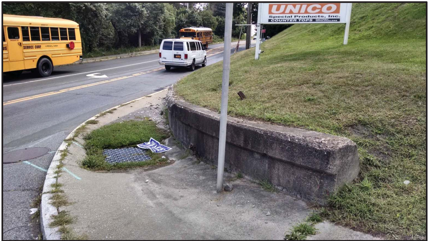
Figure No. 1: End of retaining wall at intersection of Renwick Street & Marine Drive. View looking southeast at intersection.
