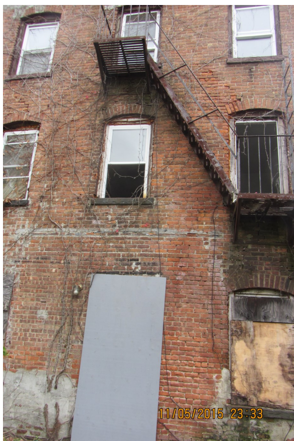
Rear of the building
