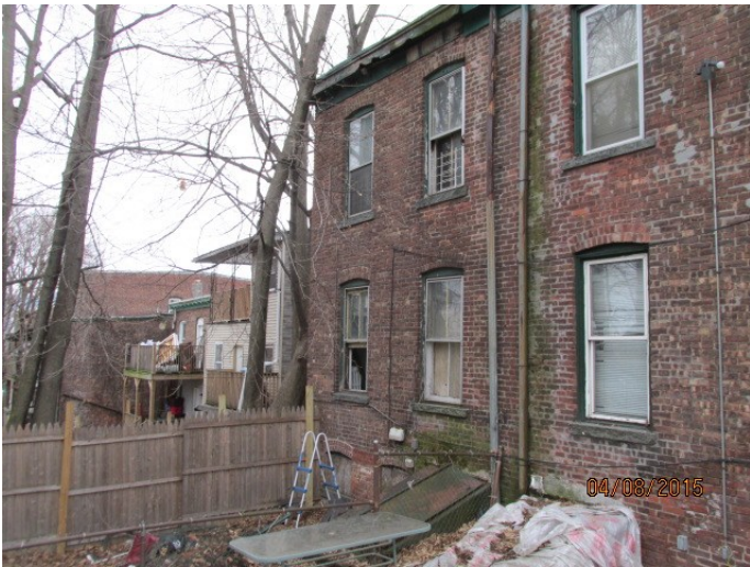
Rear of Building
