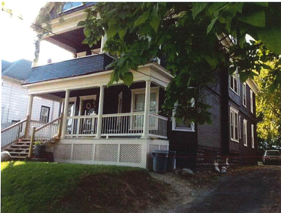
Entire Exterior repaired with new cedar siding and then, was scraped and painted.
