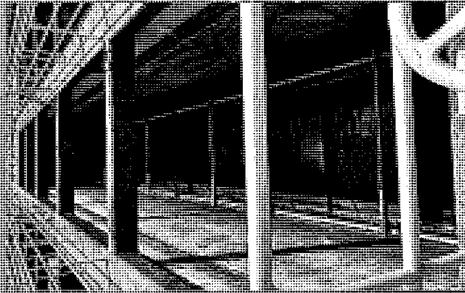
Inspecting and replacing guide flights and chain links on settling collectors of Tank # 2.
