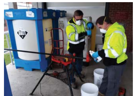
Water Department Generator Diesel Day Tank Replacement
