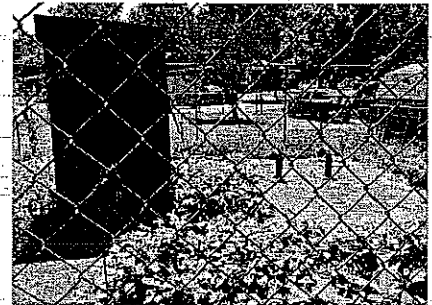
Pump Station Project Site
