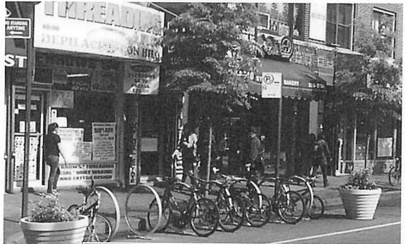
Bike corrals provide on-street parking for bicyclists, typically on major commercial thoroughfares. They include bike racks as well as bollards and/or planters which separate the space from adjacent parked cars. A bike corral can accommodate 6-8 bicycles in the same space allocated for a single occupancy vehicle.
