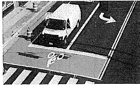
Figure 6. A high visibility bike box for turning cyclists.
