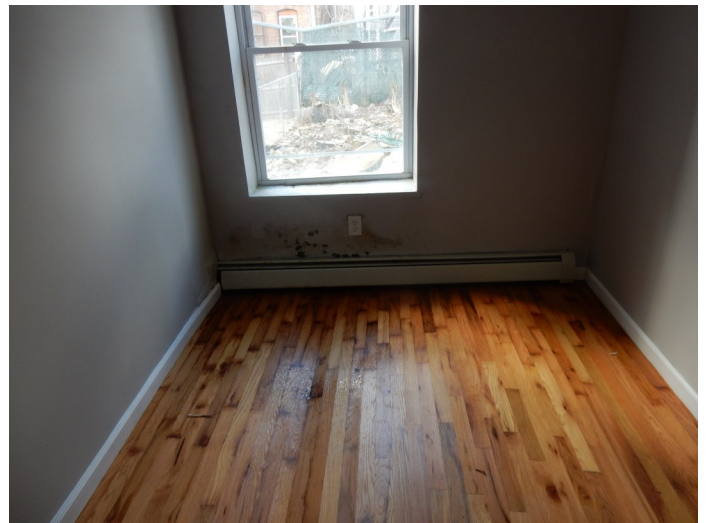
Interior Photos (above—1st floor: showing water damage to floors and wall; below—2nd floor unit)
