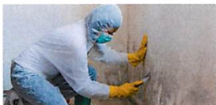
Post construction cleaning
