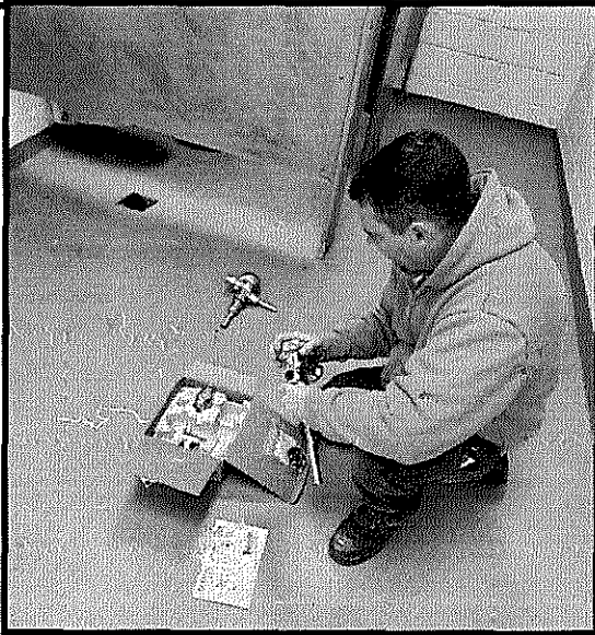
REPAIRED RECREATION DEPARTMENT BATHROOMS
