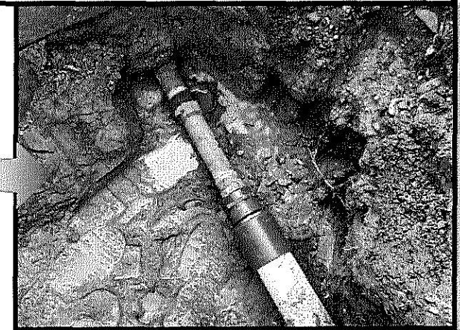
FIXED IRRIGATION LEAK AT THE DELANO-HITCH PARK
