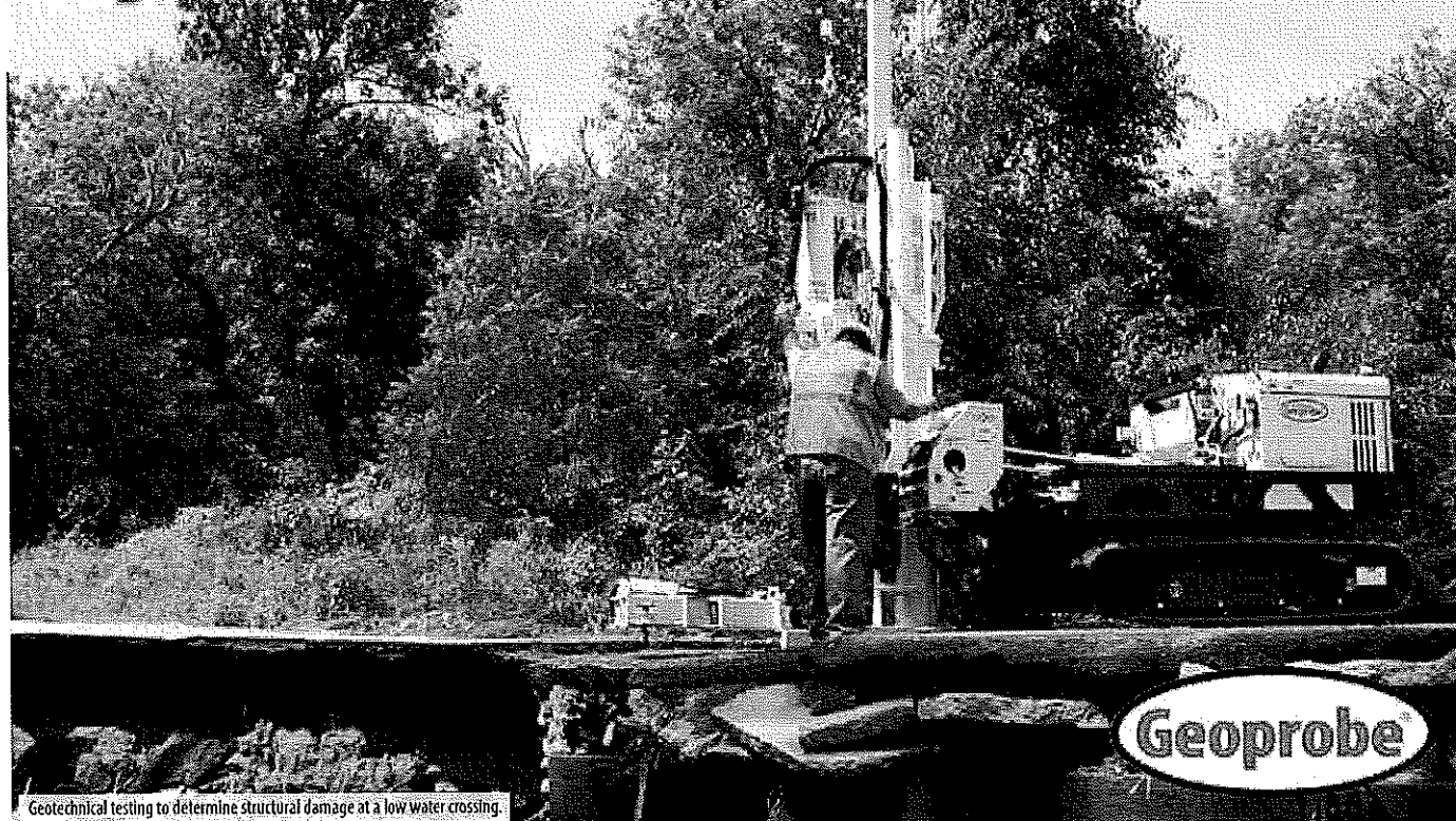
Geotechnical testing to determine structural damage at a low water crossing.
