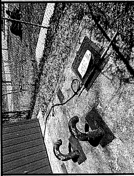
INSTALLED NEW FLOATS AT CRESCENT AVENUE PUMP STATION
