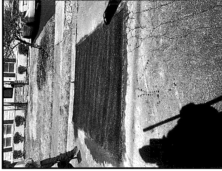
Repaired Pothole
