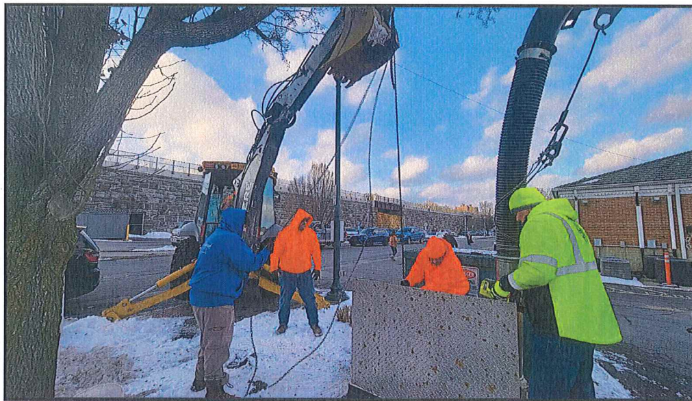
Department of Public Works staff doing emergency repairs of Front Street's sewage pump station
