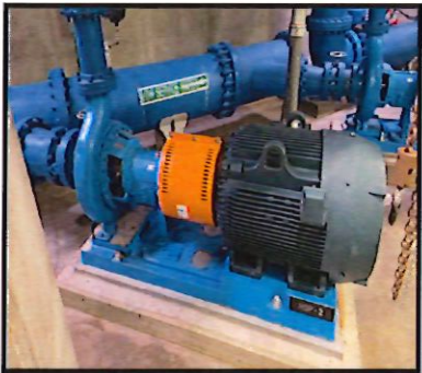
Water Department Staff Completing Repairs to the Water Pump
