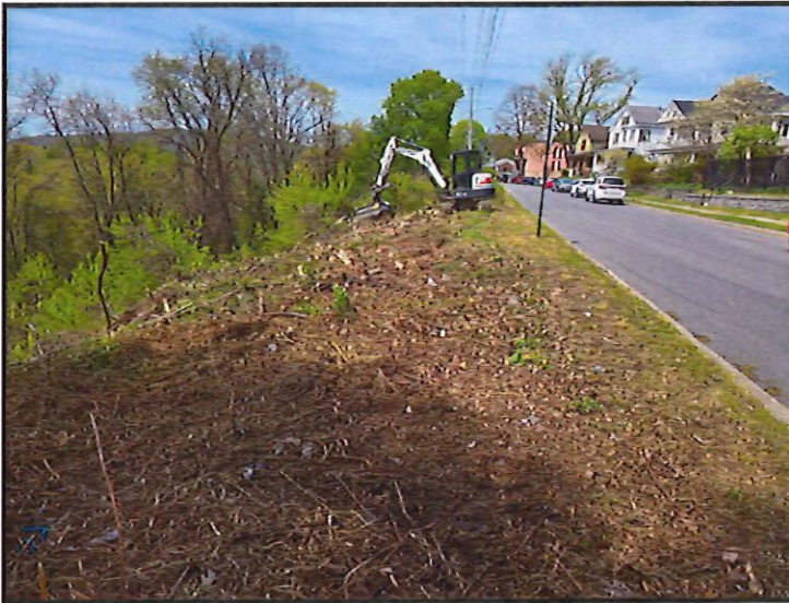
Bluff Clearing in Progress
