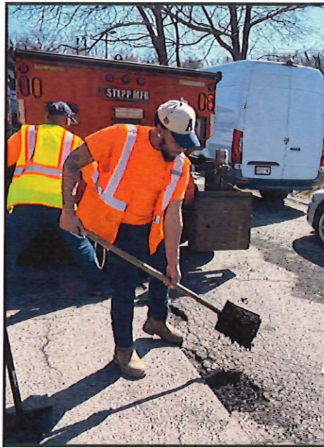
DPW Staff repairing potholes throughout the city
