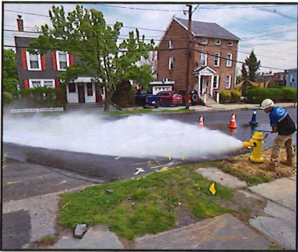
City staff flushing a fire hydrant
